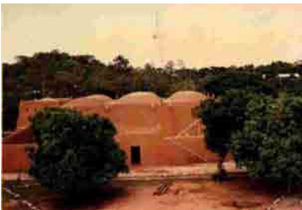
Figure 2: Traditional Architecture of the North. A structure masterly covered with several domes with very small openings on external walls. Source: Author's photograph.
