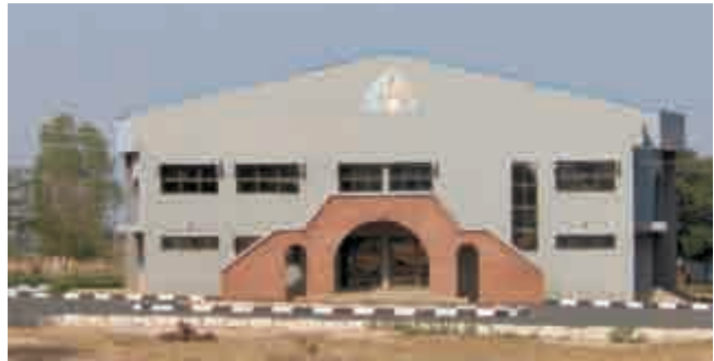
Plate 34. Multipurpose Hall, Federal University of Technology, Yola.
