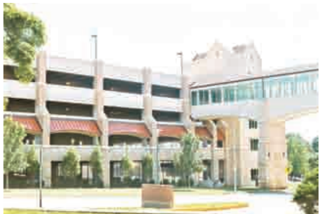
Plate 20. Multi-storey car park with bridge at the University of Missouri, Kansas City.
