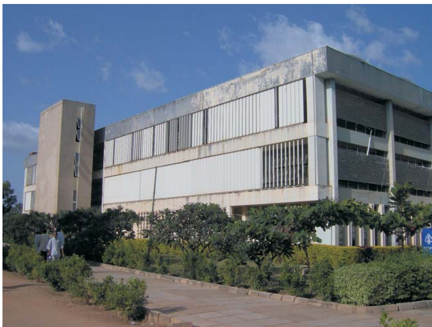
Plate 6: Kashim Ibrahim Library, Ahmadu Bello University, Zaria by Egbor and Associates. Source: Author's photograph, 2005.
