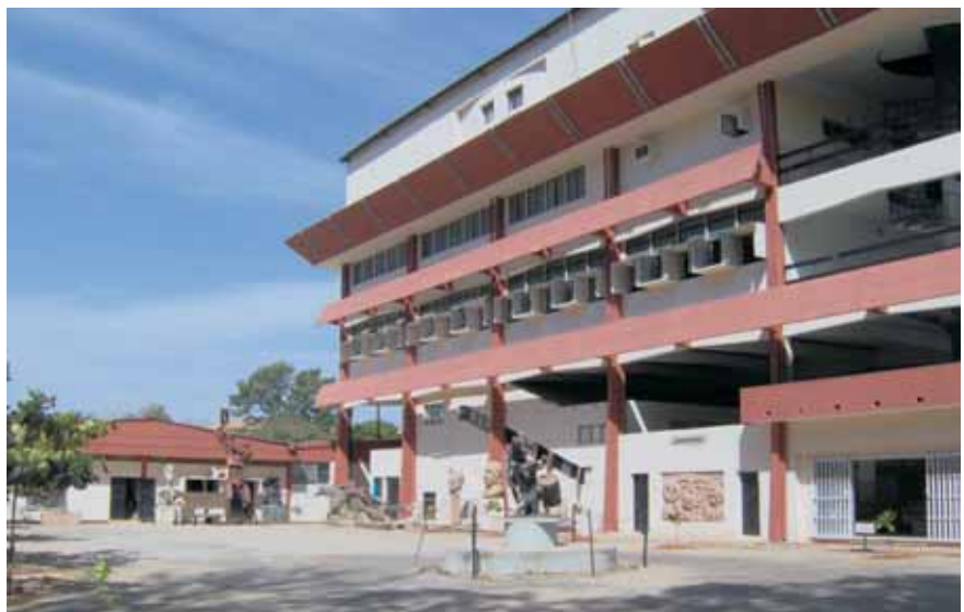
Ahmadu Bello University, Zaria. . Source: author's photograph, 2005.
