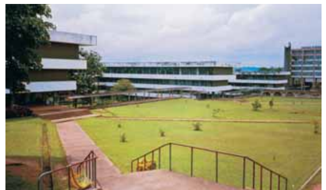
Obafemi Awolowo University, Ile-Ife. The Quadrangle with the Humanities Buildings. Source: author's photograph, 2004.
