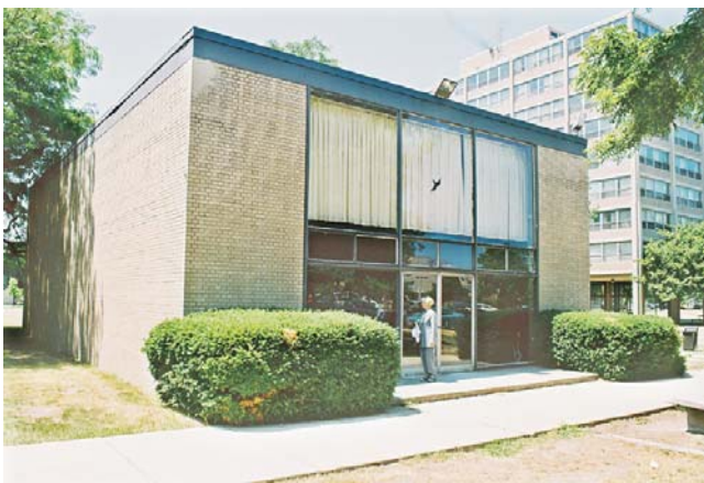
Chapel by Mies Van der Rohe at Illinois Institute of Technology, Chicago. Source: Author's photograph, 2005.
