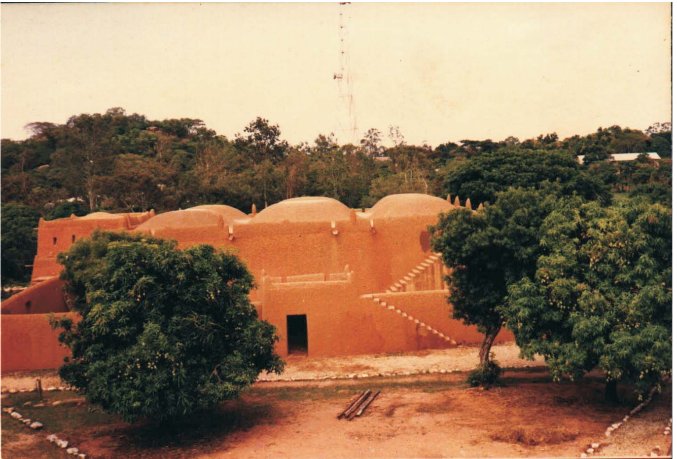
Figure 2: Traditional Architecture of the North. A structure masterly covered with several domes with very small openings on external walls. Source: Author's photograph.
