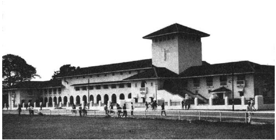
Figure 3: Colonial Style. High Court Building, Lagos, by Watkins and Partners, 1950. Source: Schultz, 1975, p.26.
