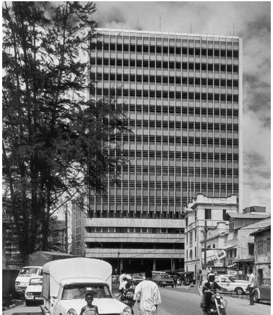
The modern style: Bookshop house in Lagos. Source: John Godwin archives.
