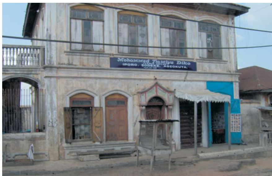
Example of the Brazillian style. A two-storey building in Abeokuta, Ogun State. Source: Autho's photograph, 2005.
