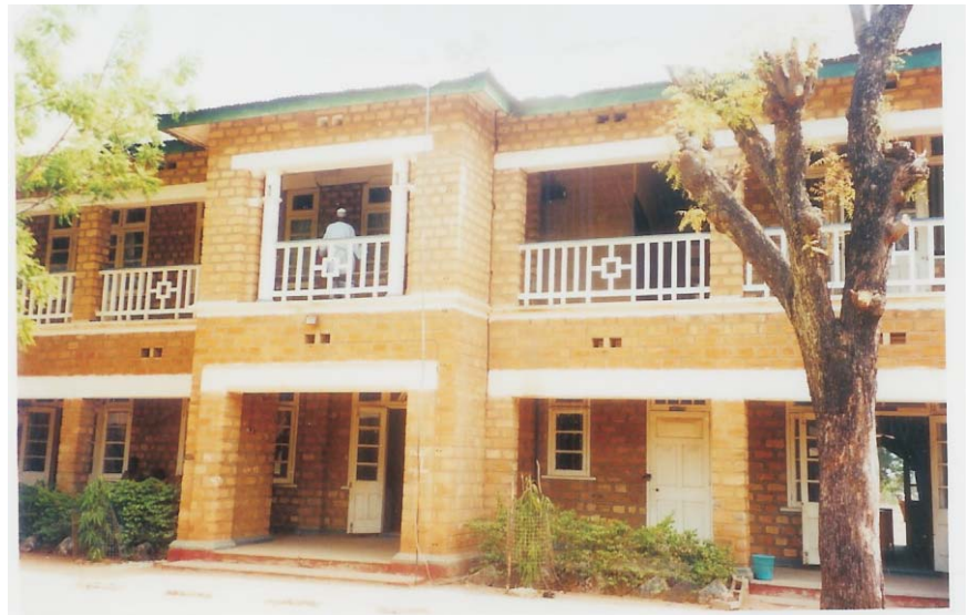
Colonial architecture: Administrative Block, General Murtala Mohammed College, Yola. Source: student assignment, 2006.
