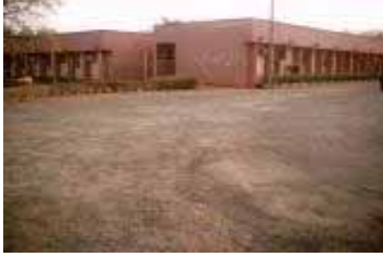
Federal University of Technology Central Administrative Block Source, Student Photograph
