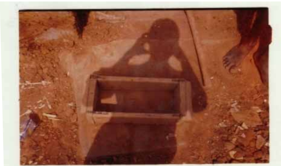
Brick form work (moli)
