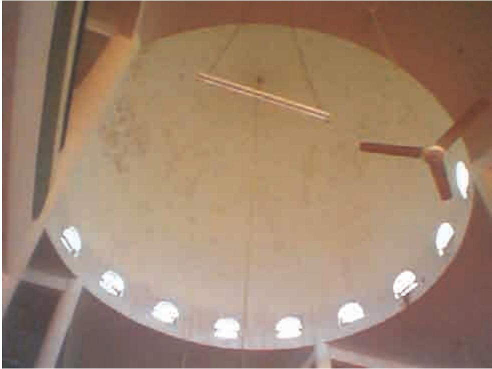
PICTURE SHOWING THE DOME FROM INTERIOR.
